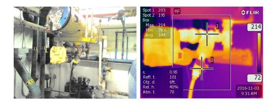
Low Pressure Steam Trap pipingOperating Temperature, \*F±235°Ambient Temperature, \*F104Insulation selectedFiberglass
